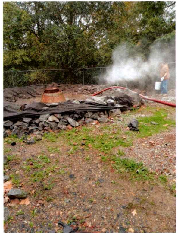
MH 1866 During Cleanup
