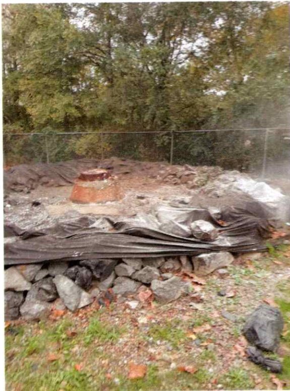
MH 1866 After Cleanup
