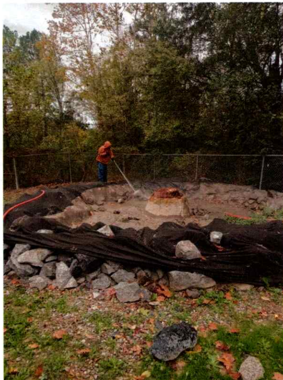
MH 1866 During Cleanup
